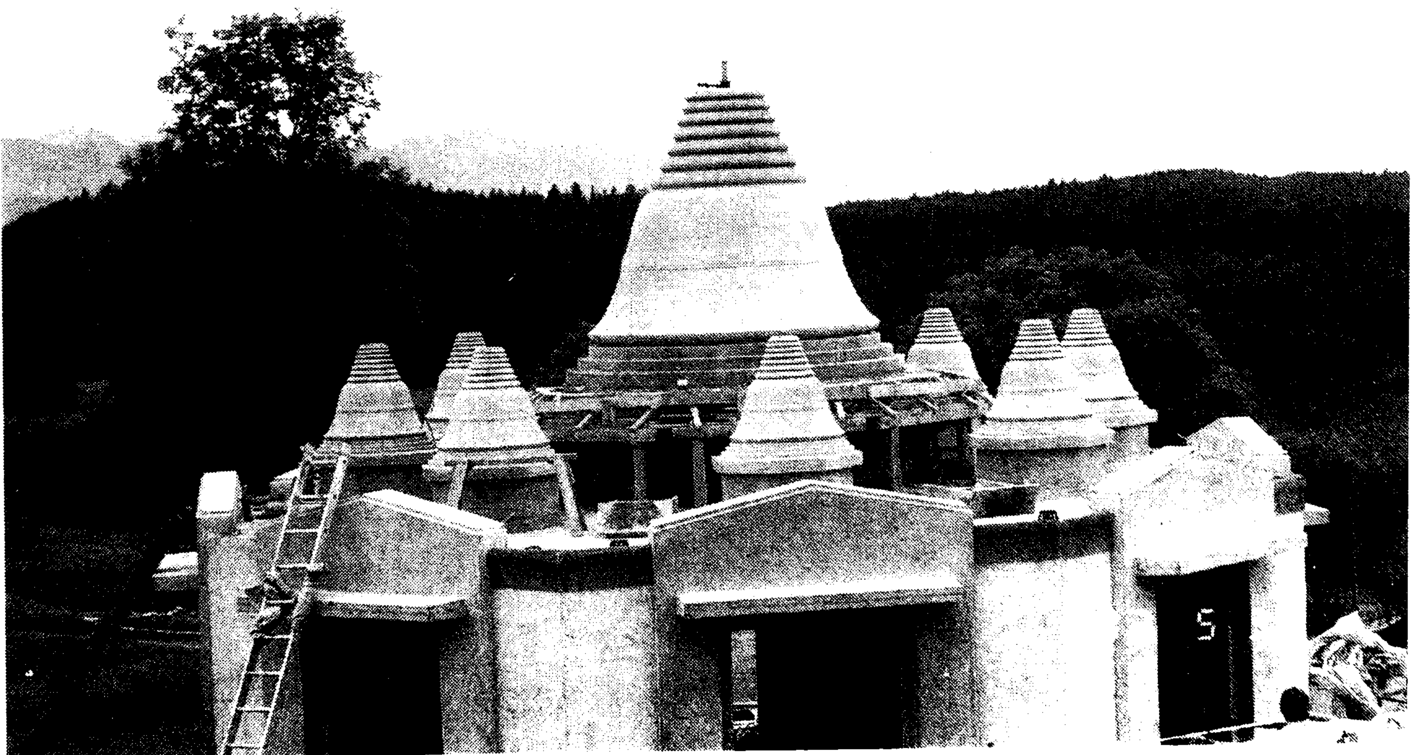
Finished main dome with the eight smaller domes (IMC-Austria)
