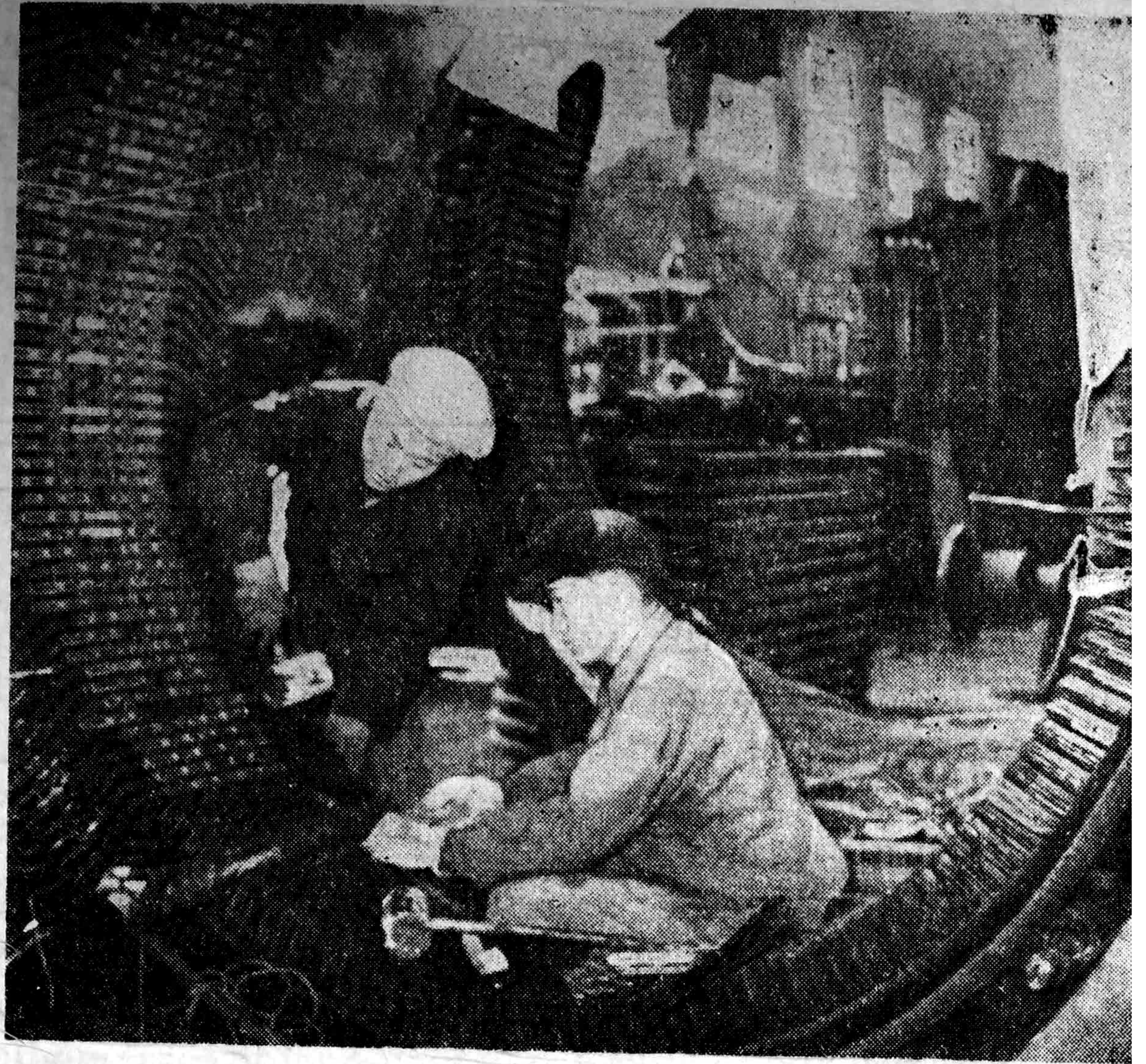
Generators being assembled at the Daian Electric Appliances Factory
