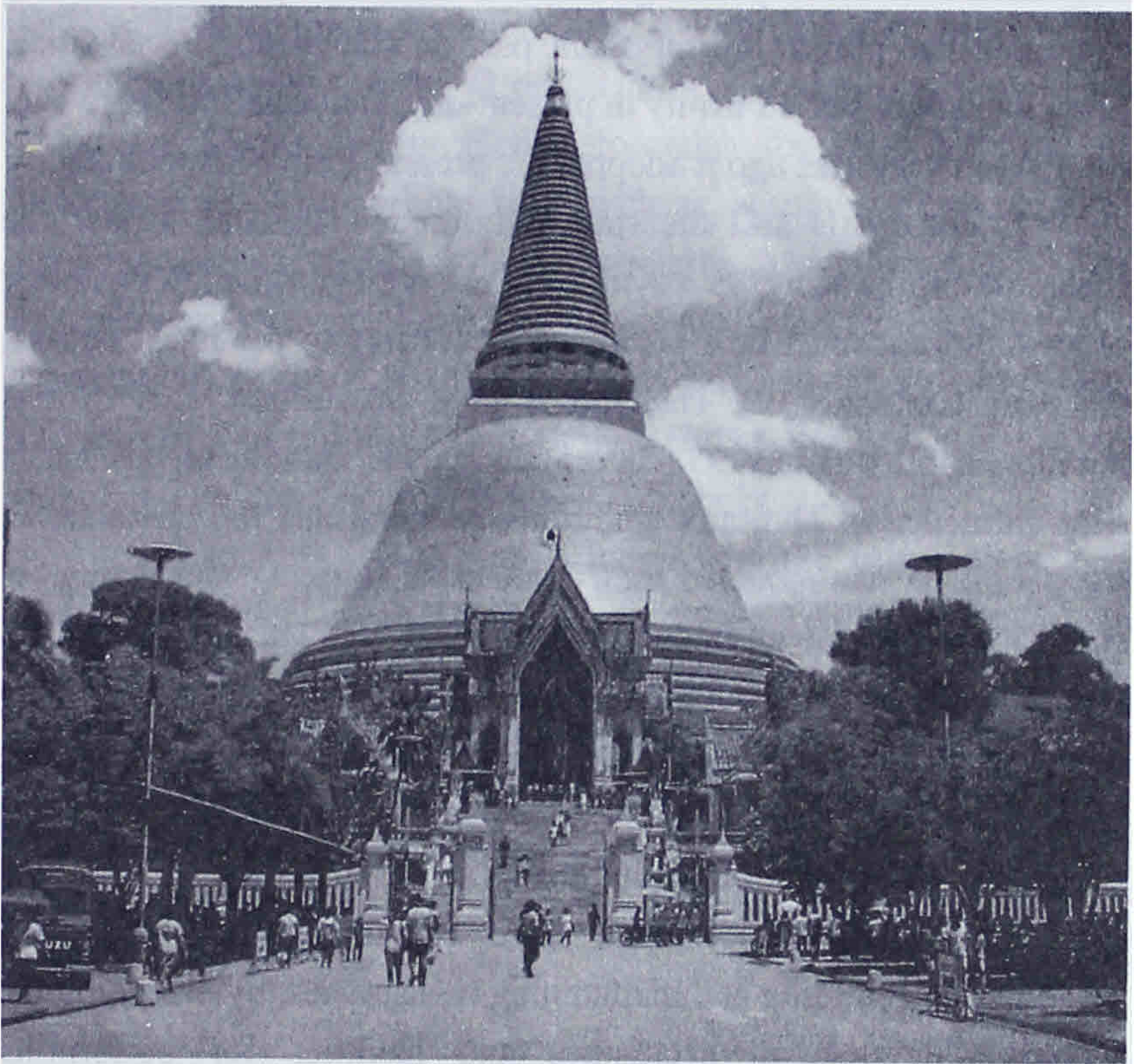
Phra Pathom Chedi at Nakorn Pathom in Central Thailand is the first stupa in the Golden Peninsula and the world's tallest Buddhist monument (127 m.), with the origin traced to Asoka's time (3rd century B.C.E.).
